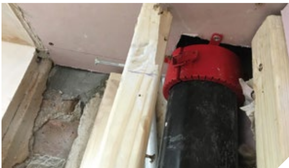
Photo 2. This internal 100mm drain penetrated the flats from the floor above (ie, a fire cell perimeter). Although this work would be hidden from view and the new fire collar was fitted, the standard of workmanship was poor. Hence, this was important to see during site visits as this perimeter of a fire compartment is exactly the kind of area that a fire would break through. A good example of something to discuss with your contractor so they remember to seal off in detail utilising, as a minimum, B1 foam and sealant.
