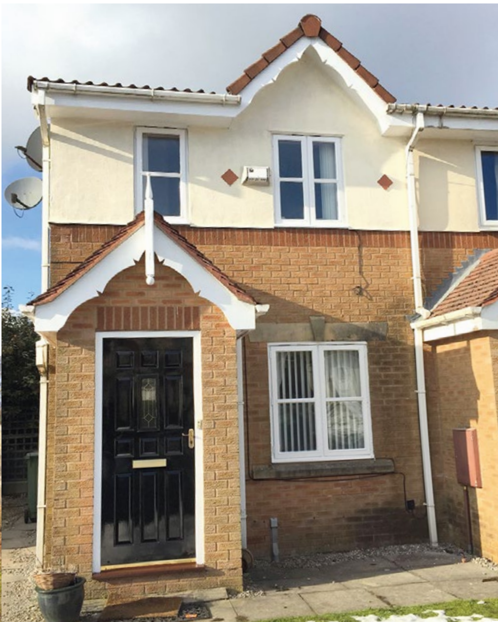
Reservoir latest development project
