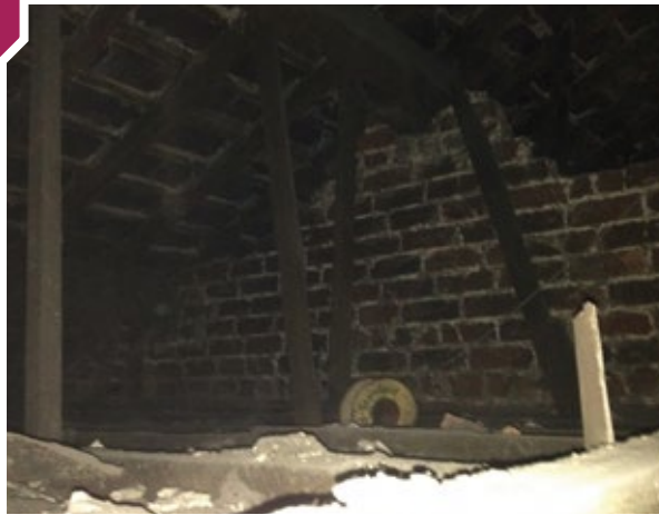
Photo 7. Victorian brick firewall in roof space, incomplete and left hanging. Property uninsurable or mortgagable. This wall was made structurally safe, extended up to the roof in block and the new double 100mm timber, fireline clad wall seen on photos 8 and 9.
