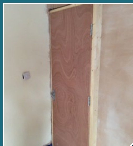
Photo 5. In this flat conversion, this FD60 front door has non-fire-rated steel handles and sits in a softwood frame built into the room, with no door closer. This door set had to be removed and a new doorway cut out to fit a correct door and frame.
