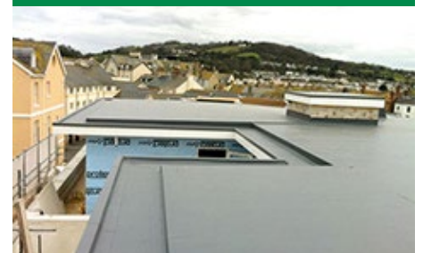
5 A new-build single-ply large span roof to block of flats
