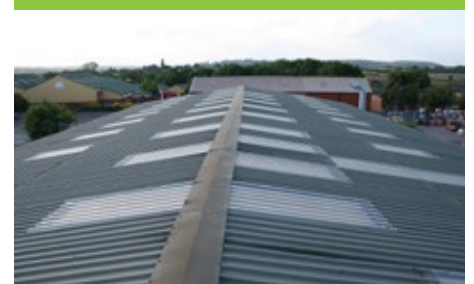
6 A new-build metal sheeted industrial roof
