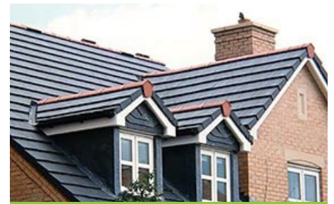
1 A new-build concrete tile roof
