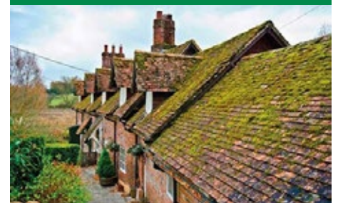
3 A 1920s-clay tile roof
