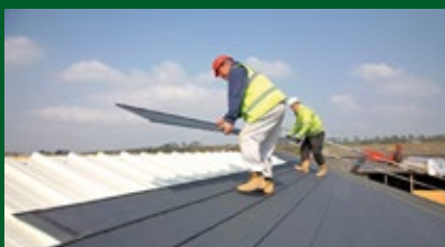
14 A steel plastic-coated cladded roof
