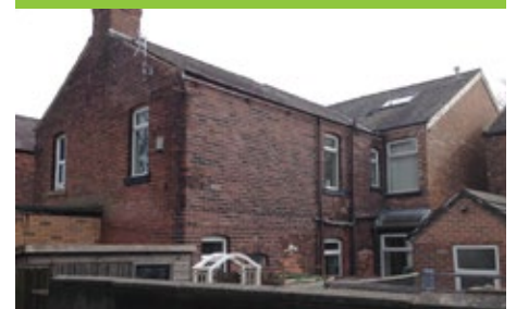
4 Victorian slate roof
