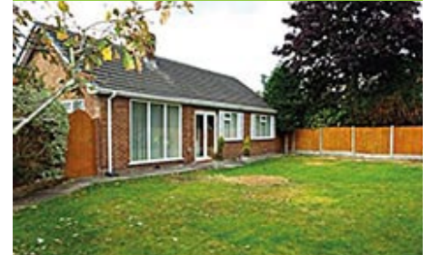
2 A 1960s-porous tile roof
