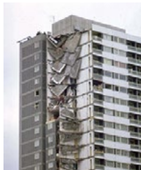
Photo 4: Ronan Point Collapse
