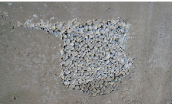
Photo 3: Concrete Consolidation
