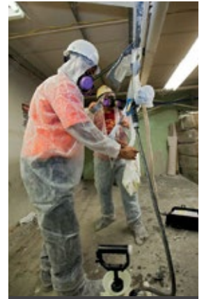
Photo 14: Typical spraying down dust & bag sealing
